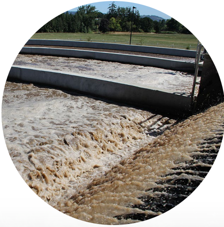
Oxidation ditch aeration basin with three zones.
