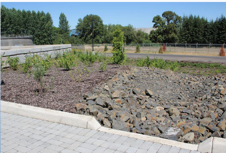
Drainage outlet for permeable paver system
