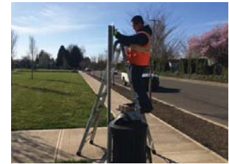
Carlos Ochoa – Street Crew (5 years) – Installing new signage
