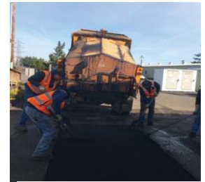
Street crew paving
