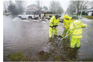
Kristine Reed, right, Parks Maintenance (13 years), clearing storm drain during December 2015 rains.
