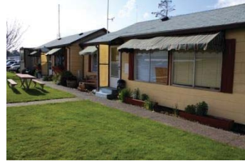
FBO building will be demolished in the summer of 2016
