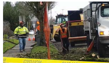
Jeff Hendricks, left, Parks Maintenance (11 years), removing hazardous tree at the Chamber of Commerce.
