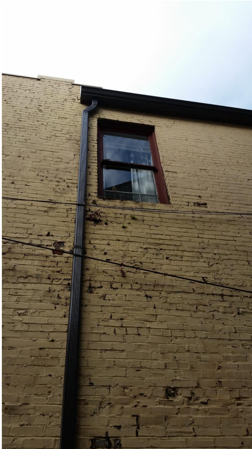
ALLEY EXTERIOR SHOWING THE EXISTING COLOR AND CONDITION OF THE BRICK
