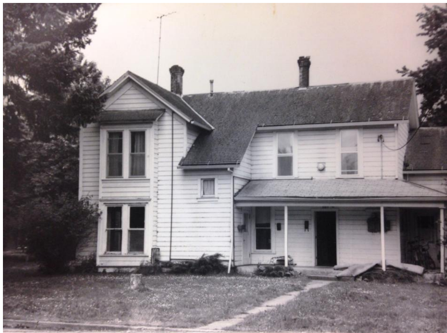
Original 1983 Survey Photo
