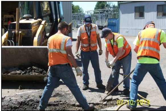
Street Crew Pavement Repair Training
