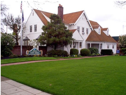
McMinnville City Hall
