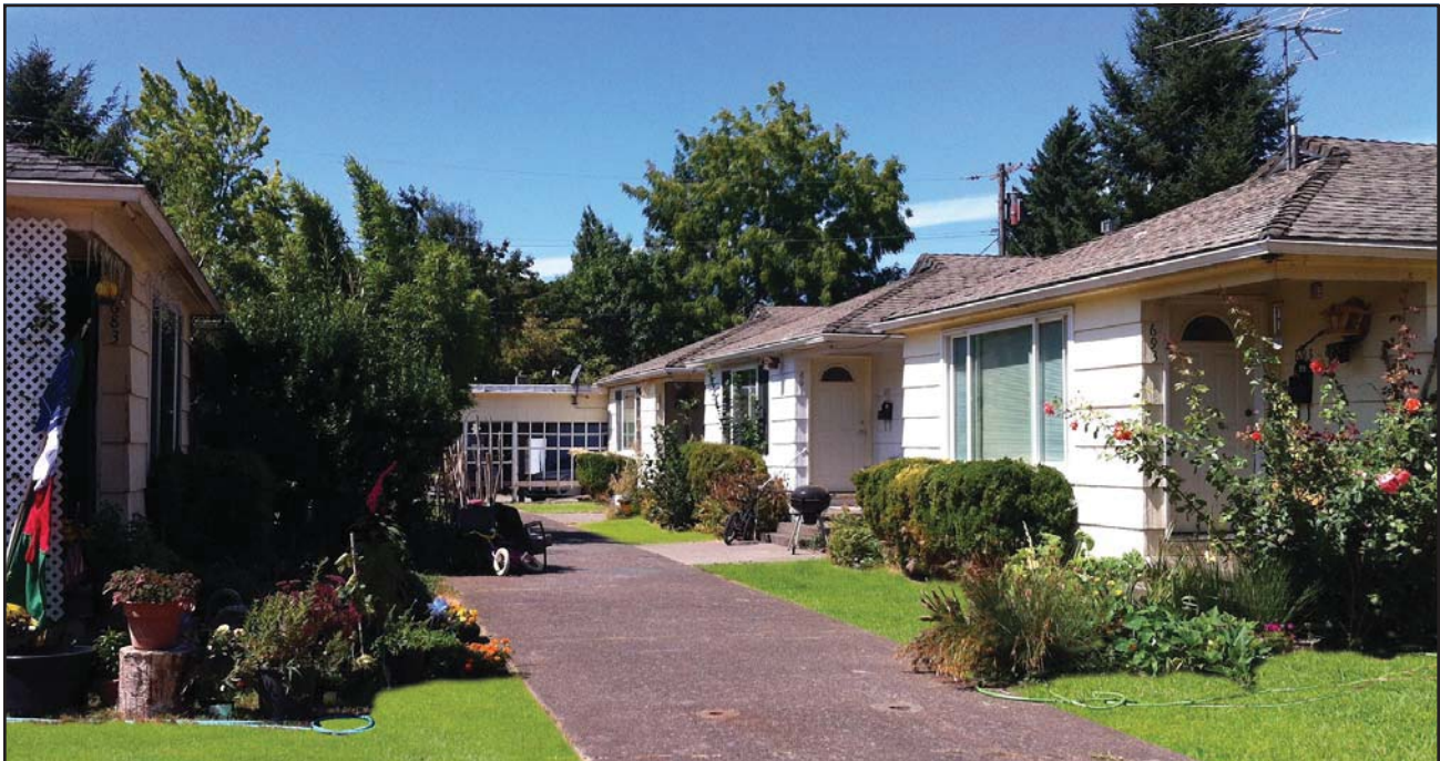
The Catterlin Cottages in Salem, OR, are six detached one-story homes, each approximately 38'x24', fronting onto a central courtyard.
