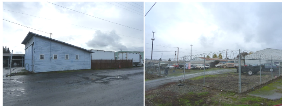
Under-development in the area
