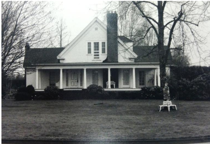
Original 1983 Survey Photo
