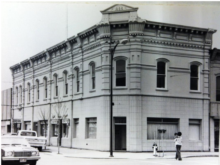
Original 1983 Survey Photo
