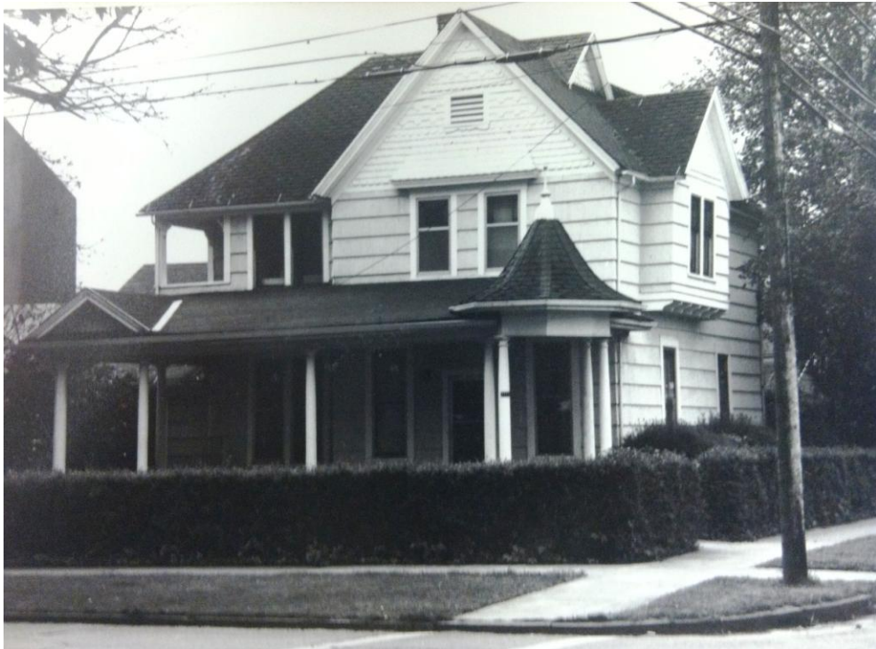
Original 1983 Survey Photo
