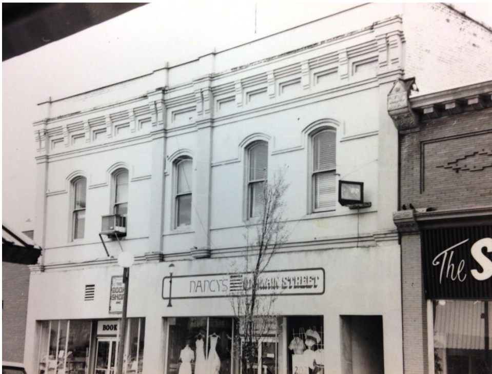
Original 1983 Survey Photo
