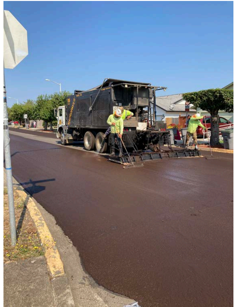
SLURRY SEAL APPLICATION
