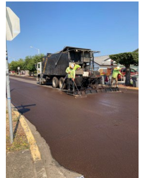
Slurry Seal Application
