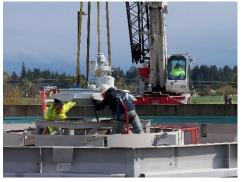
A crew from Stettler Construction uses a crane to install a drive assembly into secondary clarifier #3.
