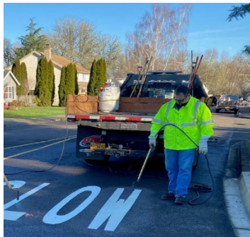
Bud Martino, UW II installing pavement markings on Wallace Road
