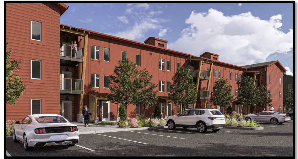
Concept plans of Stratus Village, a 175 unit affordable housing complex serving households of 60% area median income or less.
