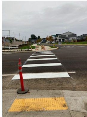
Rapid Rectangular Flashing Beacon crossing installed by Street crew
