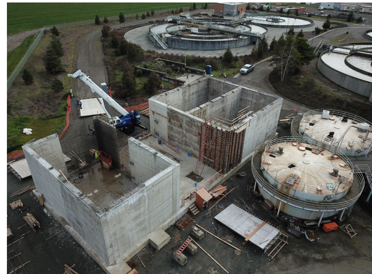
The City continues to invest in upgrades to the public sanitary sewer system in 2024-25 by addressing solids capacity issues with upgrades to our solids handling processes.
