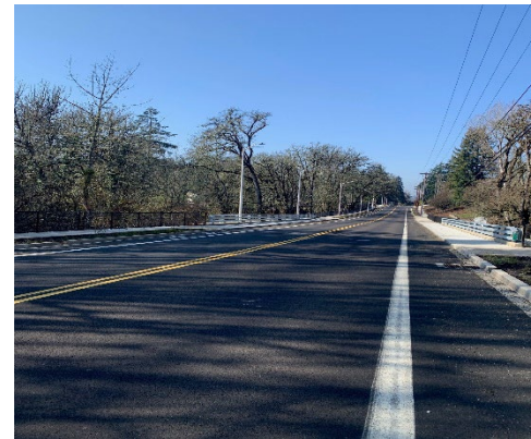
In early 2021, the $4.8-million Old Sheridan Road Improvements project was completed, improving vehicular, pedestrian, and bicycle safety between SE Cypress Lane and Highway 99W. This project was the last of the five major Capital Improvements identified in the transportation bond measure approved by the voters in 2014.
