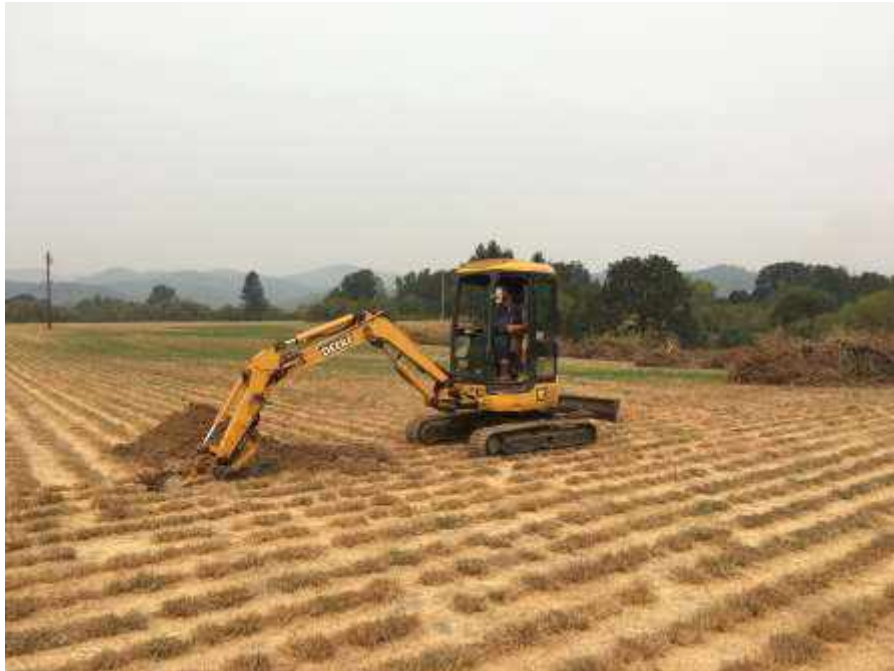
Test Pit TP-5, Facing Northwest, Looking at Western Portion of Site
