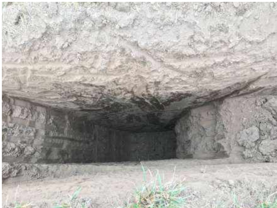
Test Pit TP-15
