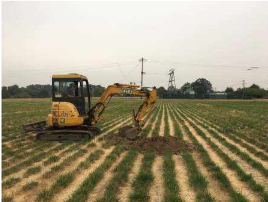
Test Pit TP-15, Facing South
