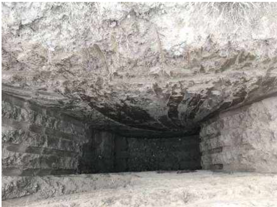
Test Pit TP-2
