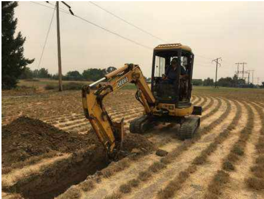
Test Pit TP-8, Facing South
