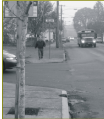
Sidewalks and Curb Ramps on Baker Street
