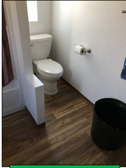
Toilet & Floor After
