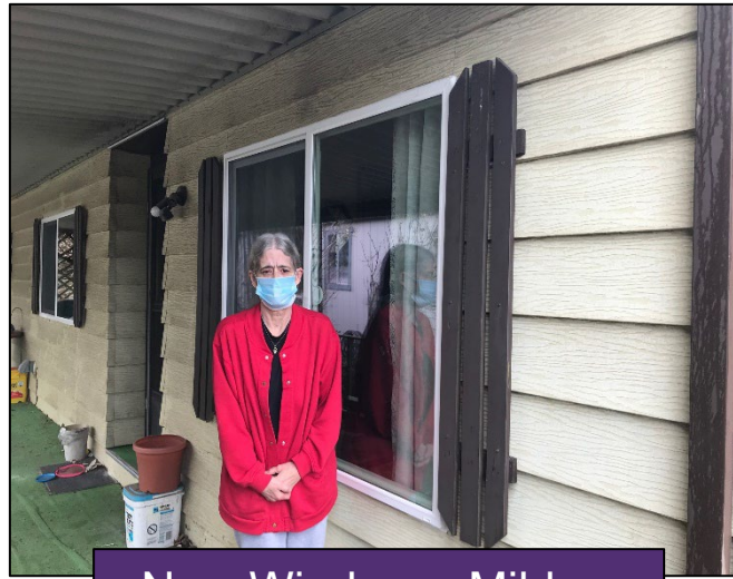
New Windows, Mildew Abatement, Dry Rot Repairs
