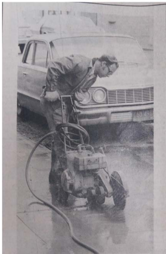
DE-PAVING THE WAY -- Trees are being planted throughout the downtown area this week as part of Committee on Redevelopment beautification plans. That work follows last week's efforts by Don Stapleton, employee of Jack Squires Construction, pictured above with sidewalk cutter making necessary cuts for curbside planting areas. Other work downtown this week includes undergrounding of utilities, which is closing off two blocks at a time of Third Street and is progressing at the rate of about one block per day.
