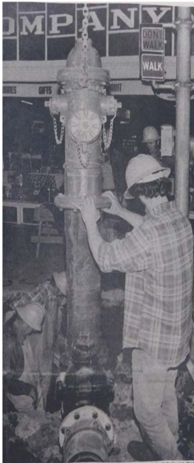
NEW HYDRANTS -- As part of the downtown work this week members of city water and light crew replaced a number of fire hydrants with those such as pictured above, which have larger water outlets. Work being done above is at Third and Ford Streets at about 11 p.m. Wednesday.
