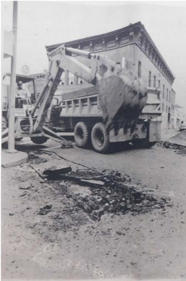
WORK BEGINS — Jeff Kizer of Kizer Excavating ears up Third Street, making way for drainage system as initial work in downtown improvement for McMinnville. Work started Monday, after many months of work by Committee on Redevelopment and
