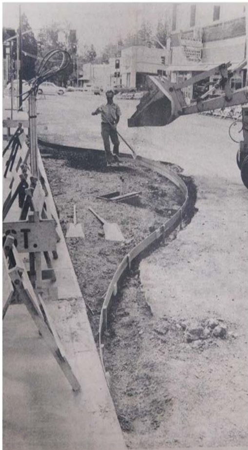
THIRD STREET ISLANDS -- Concrete forms are set in place for the curved islands which will be located in each block along Third Street. The COR beautification program for Third Street will include trees, benches, sections of new sidewalk and, at the end, a new overlay of Third Street.
