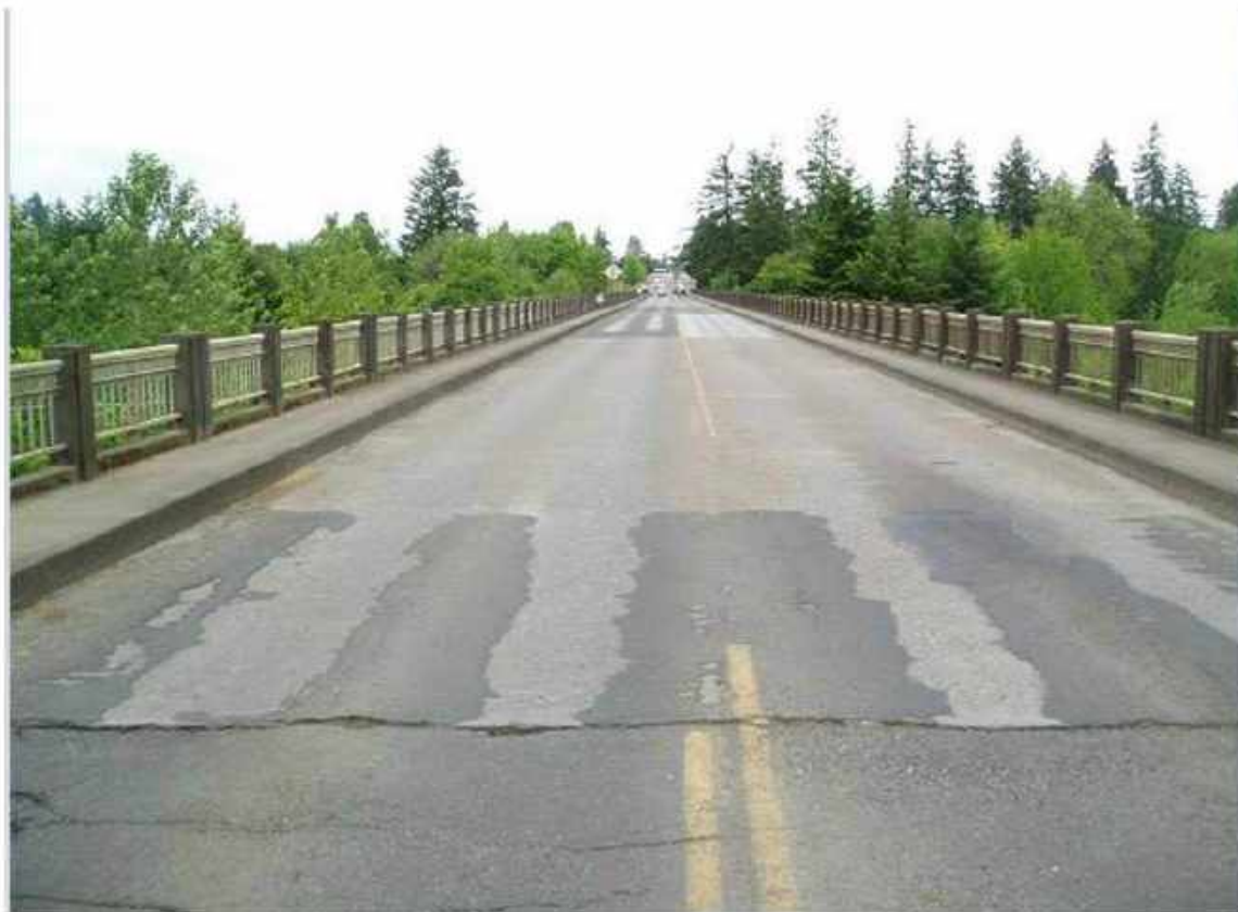
Existing South Yamhill River Bridge - Three Mile Lane, McMinnville
