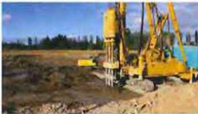
*The soils at the reservoir site are highly susceptible to seismic-induced liquefaction and required extensive deep soil mixing techniques to build a seismically-resilient facility.*
