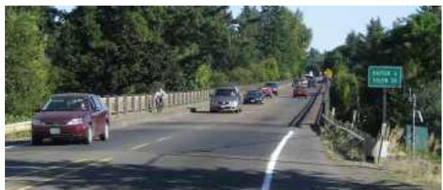
Limited Sidewalk Width on Yamhill River Bridge
