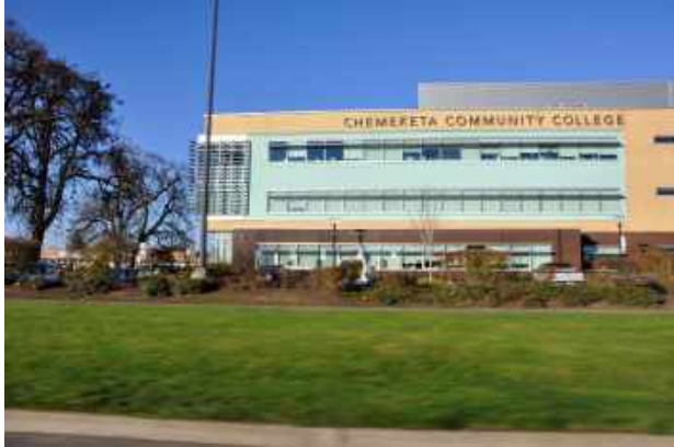
Central Neighborhood and CCC Area
