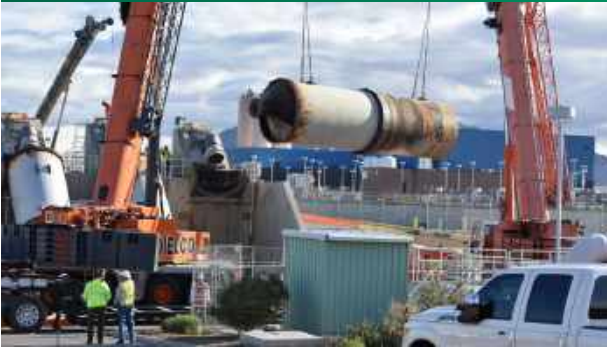
Decommissioning of the former WWTP.
