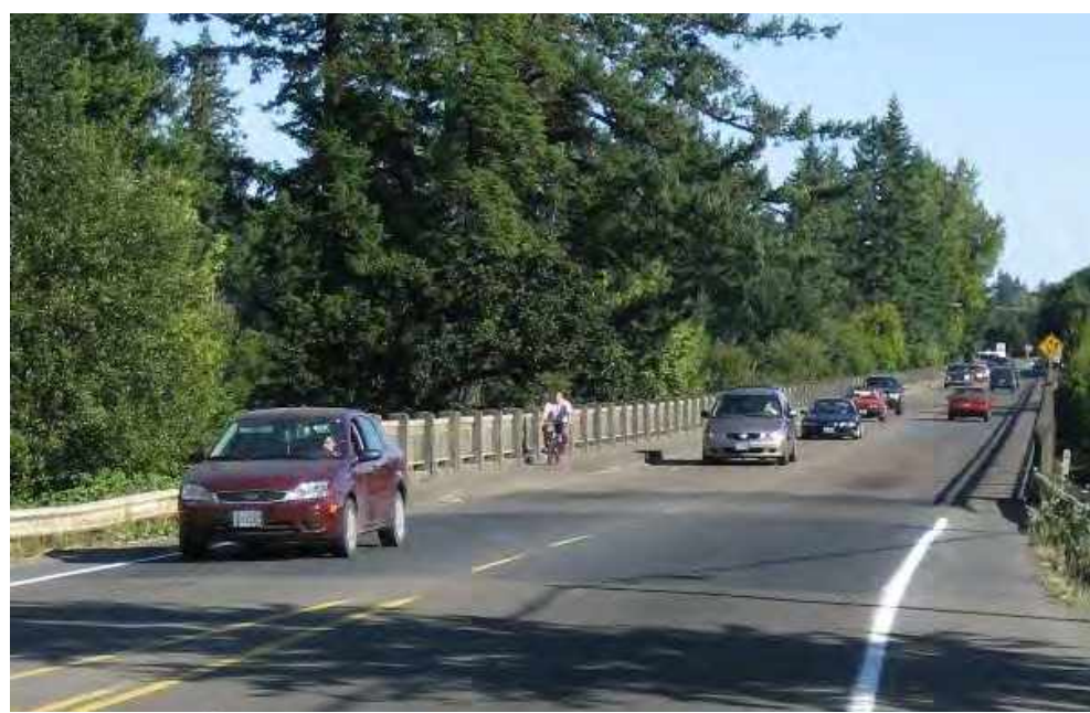
Narrow sidewalk, no bike lanes on Yamhill River Bridge
