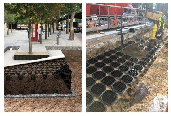
**Soil Cells** can promote root growth below paving by providing trees more space and uncompacted soil
