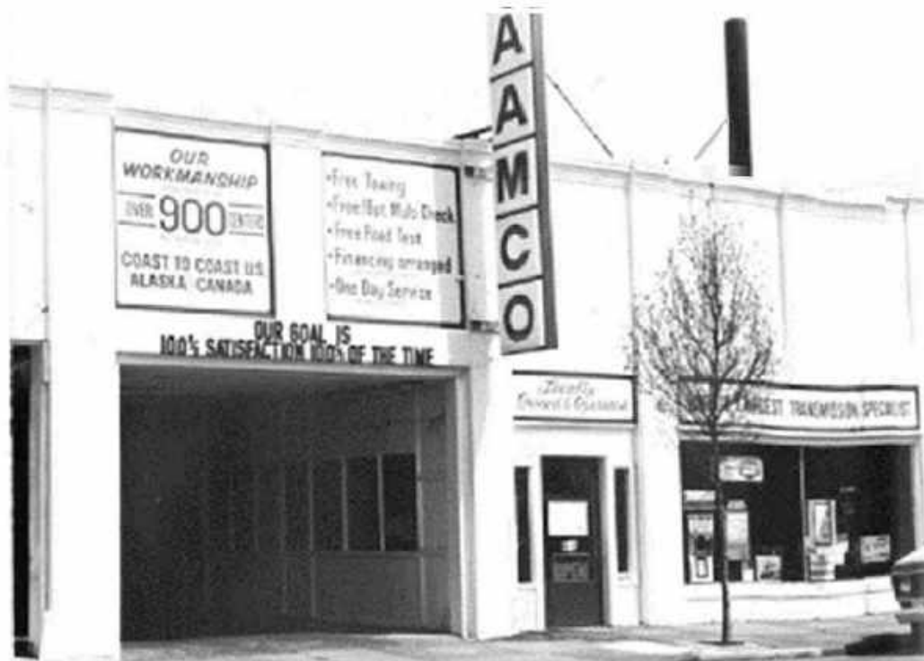
By the time of this 1983 historic survey photograph, the window to the east of the double-wide opening had been converted to an entry and the windows in the two easternmost bays had been replaced with a storefront window spanning both bays (Historic Resources Survey, City of McMinnville, Yamhill County, Oregon).
