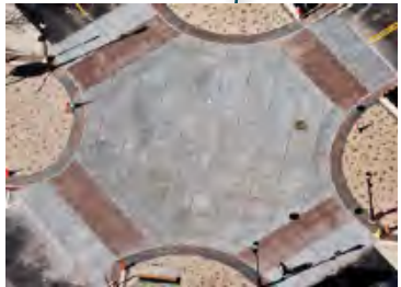
Concrete intersections with angled scoring
