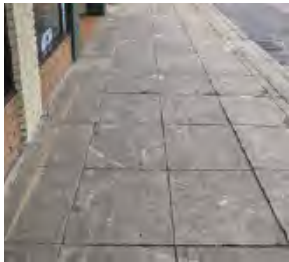
Concrete sidewalks with 2'x2' scoring
