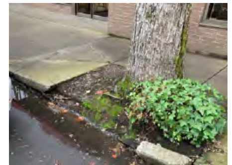
At ground-level, one can see how constrained the root systems are for the existing trees - and the damage they have caused to sidewalks and curbs.
