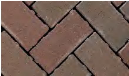
Mid-block curb extensions with permeable red clay brick pavers
