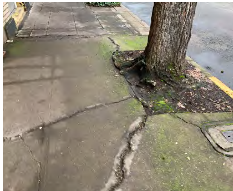
Many of the sidewalks along Third Street have been damaged by tree roots.
