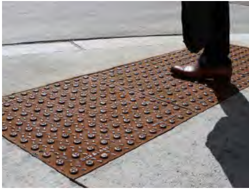
LEFT: Third Street's detectable warning surfaces (found at all crosswalks) will be uncoated cast iron.
