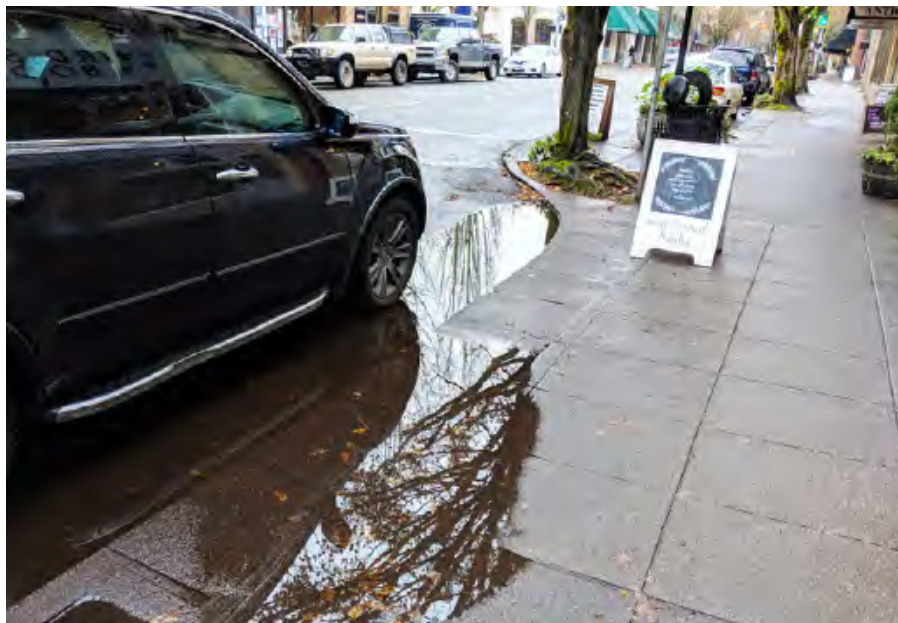
Third Street's today experiences significant ponding on rainy days. The storm sewer, like much of the street's existing infrastructure, is in need of replacement.
