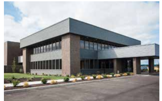
Existing office building
