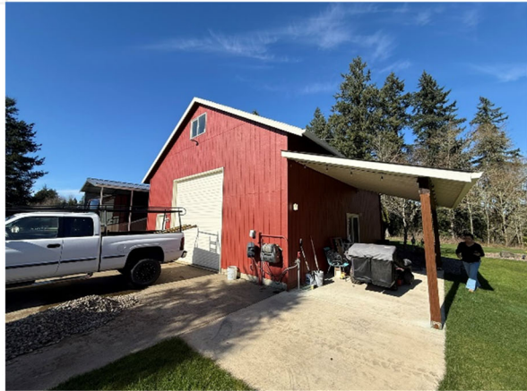
Photo #16 Permitted Shop/ADU on TL 690, facing northwest
