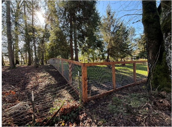
Photo #20 NE corner TL 890, facing south
