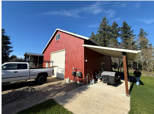
Photo #16 Permitted Shop/ADU on TL 690, facing northwest
