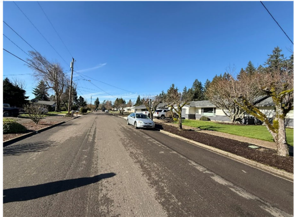
Photo #28 View along NW 25th St facing west
