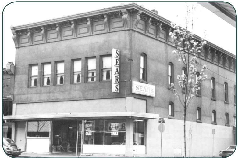
Hodson Building. Source: Primary Resource Form 173. Historic Resources Survey, McMinnville.
