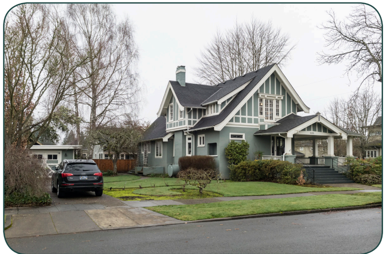
Rear south and front east facades.
