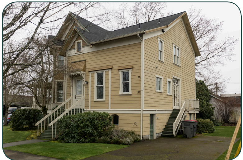
Rear west and side north facades.
