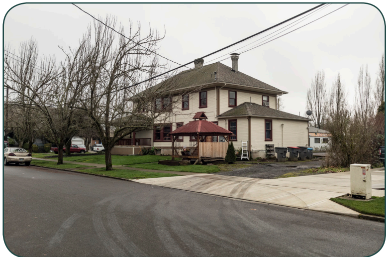
Side, north and rear west facades.
