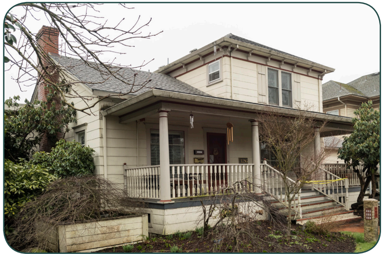
Side east and front north facades.
