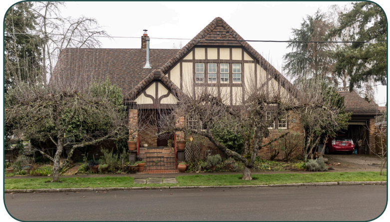
Front, south facade.
