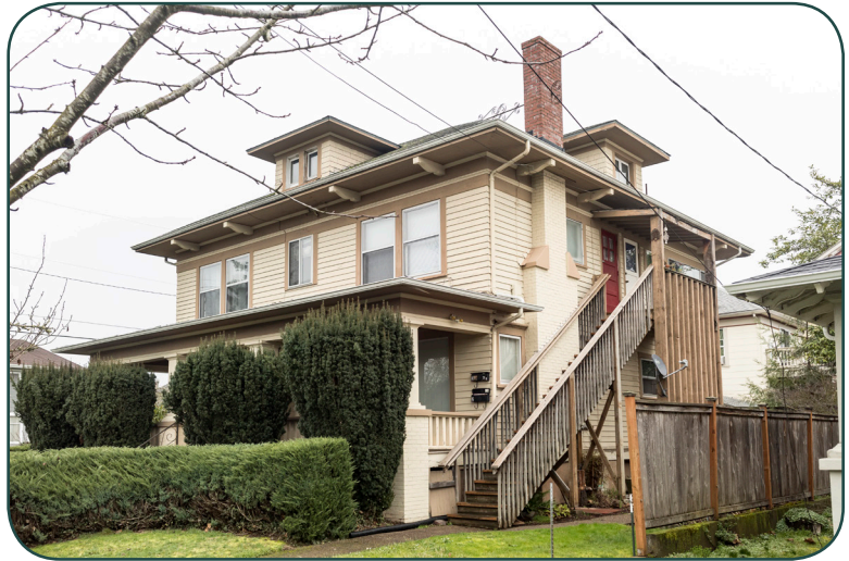
Front west and side south facades.
