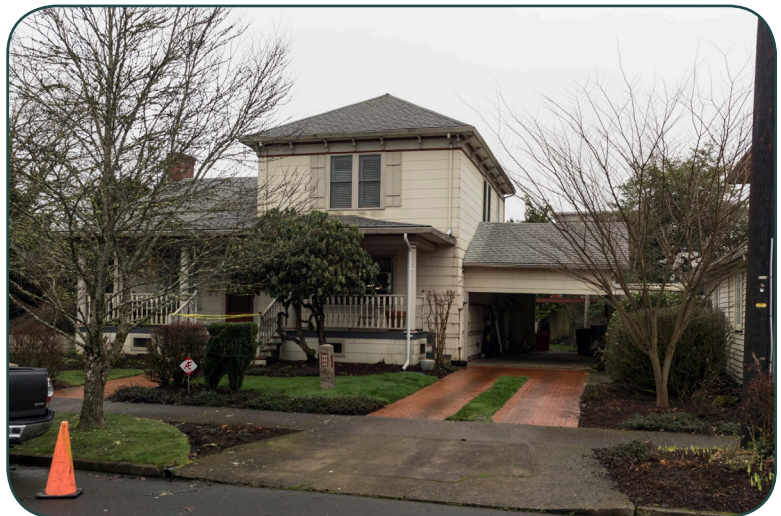
Front north and west side facades.
