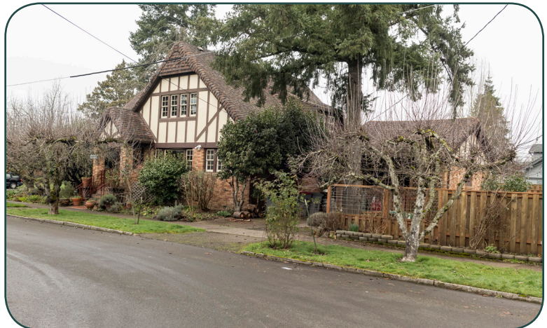
Front south and rear east facades.
