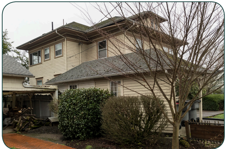
Rear east and side north facades.
