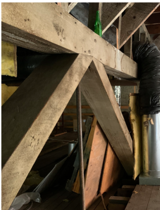
Figure 1 - Existing beams from #609.
