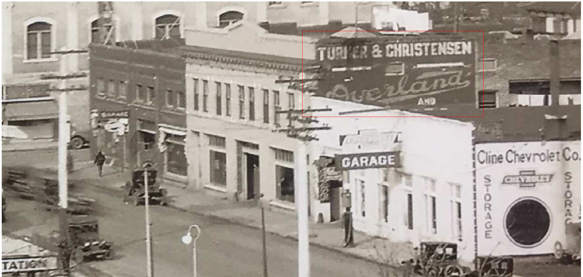
Attachment 7, 609, 619, and 641 NE 3rd Street, McMinnville, 1927
