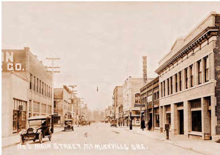
Original Structure, circa 1919
