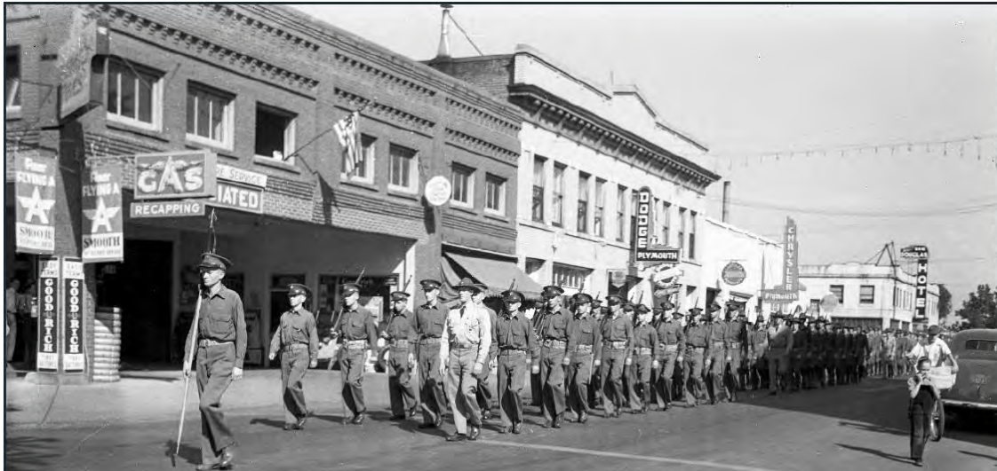
1940 Photo of 611 NE Third Street showing parapet, decorative brick work, second floor fenestration pattern, and ground floor storefronts for the garage. (Yamhill County News Register)
