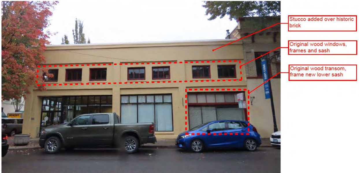
South Elevation facing NE Third Street, illustrating original features (ARG, October 2022).
