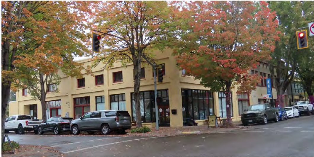
The bays at the corner of the ground floor have been infilled with the current street-facing storefront; three original storefront bays remain (ARG, October 2022).
