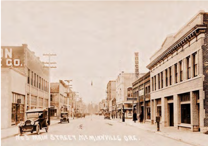
Original Structure, circa 1919
