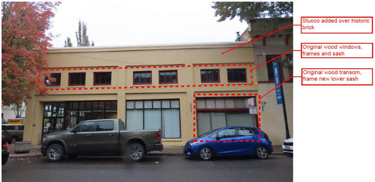
South Elevation facing NE Third Street, illustrating original features (ARG, October 2022).
