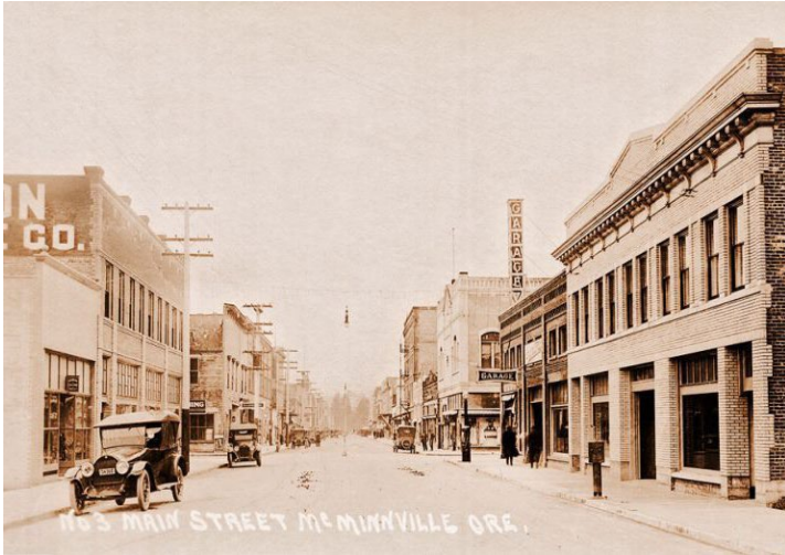
Original Structure, circa 1919
