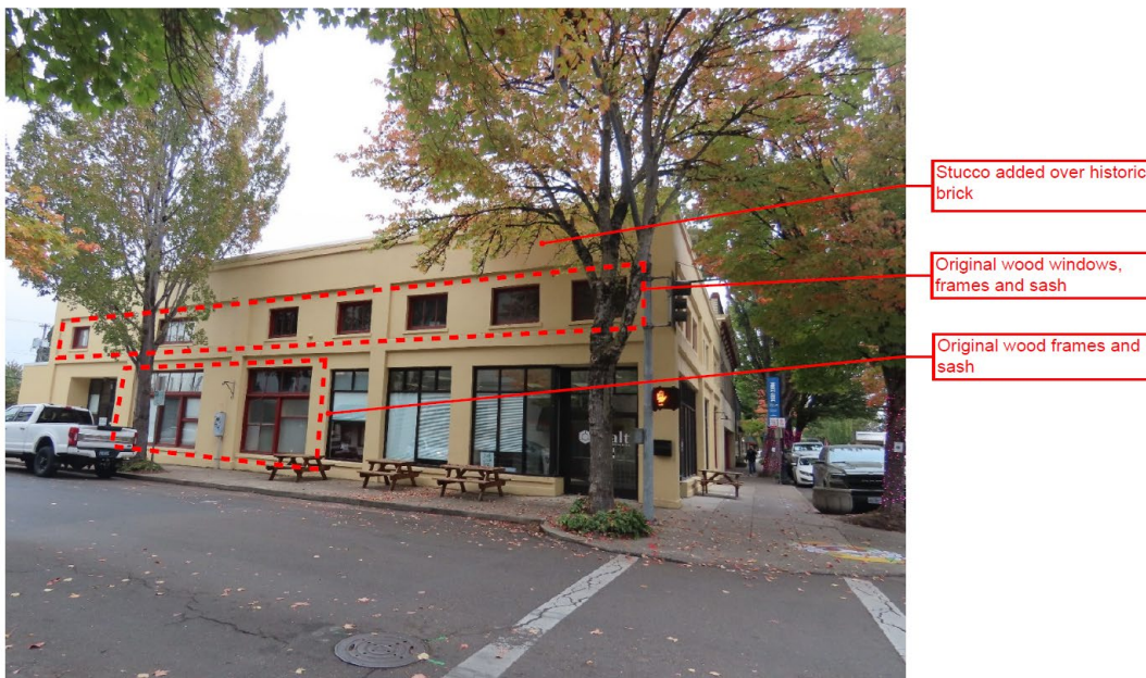
West Elevation facing NE Ford Street, illustrating original features (ARG, October 2022).
