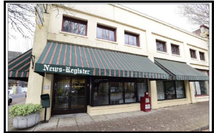
2018, Photo of 609 NE Third Street, shows the modified corner storefront filled in with a street facing storefront.
