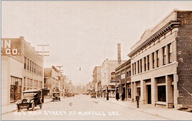
Circa 1919 Photo of 611 NE Third Street depicting two-story brick construction with a decorative parapet and extensive brick corbeling.
