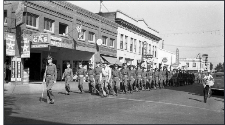
1940 Photo of 609 NE Third Street showing modified corner storefront for the gas pumps. (Yamhill County News Register)
