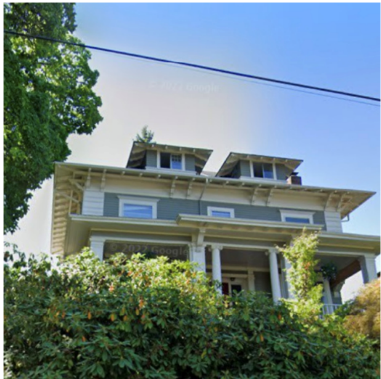
H. C. Fenton House 1705 NW 23rd Ave. Portland OR
