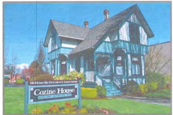
The Historic Cozine House after restoration
