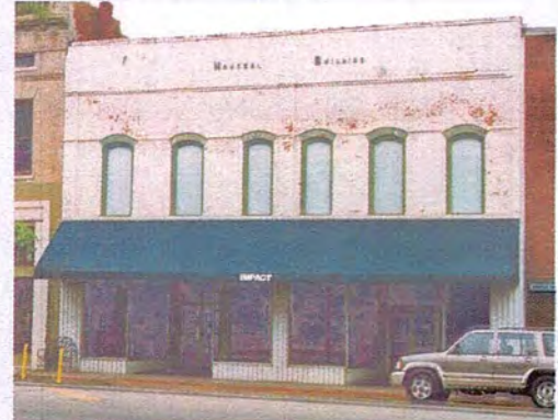
The photograph above shows the building described in the sample application prior to the rehabilitation work. Below left, the building is shown after its successful rehabilitation.
