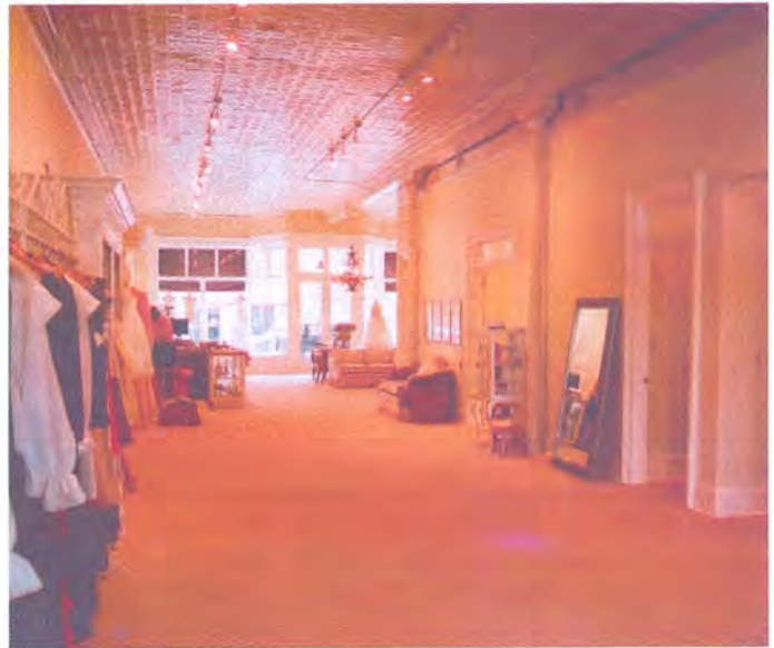
Retaining historic character: The historic tin ceiling was retained during the rehabilitation for this Main Street clothing store.
