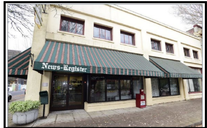
2018, Photo of 609 NE Third Street, shows the modified corner storefront filled in with a street facing storefront.
