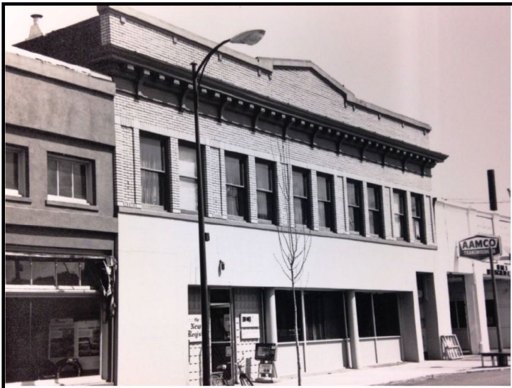
1983 photo of the property shows the modified ground floor storefronts, but with the retention of the original brickwork, parapet and second floor fenestration pattern, (Historic Resources Survey, City of McMinnville, Yamhill County, Oregon)
