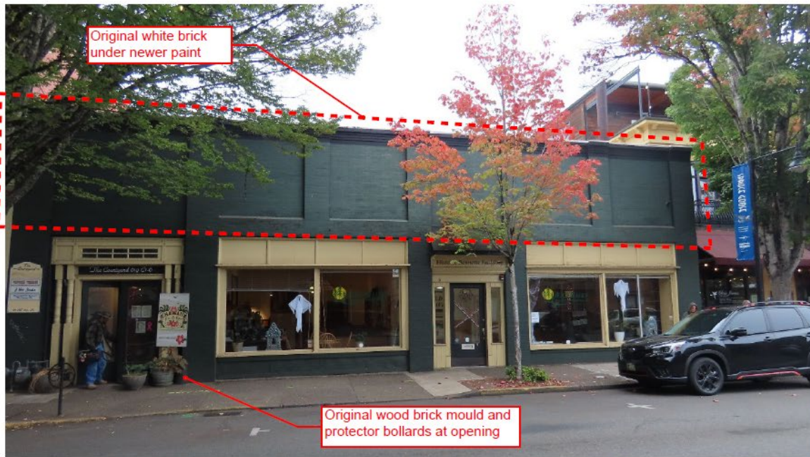
Current view of 619 NE 3rd Street (ARG, October 2022). Paired doors with wood trim elements have been inserted into the westernmost bay, while the formerly double-wide opening has been replaced with a storefront window matching the window in the easternmost bays.
