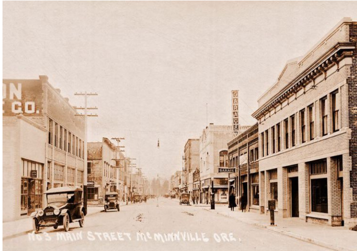
Original Structure, circa 1919
