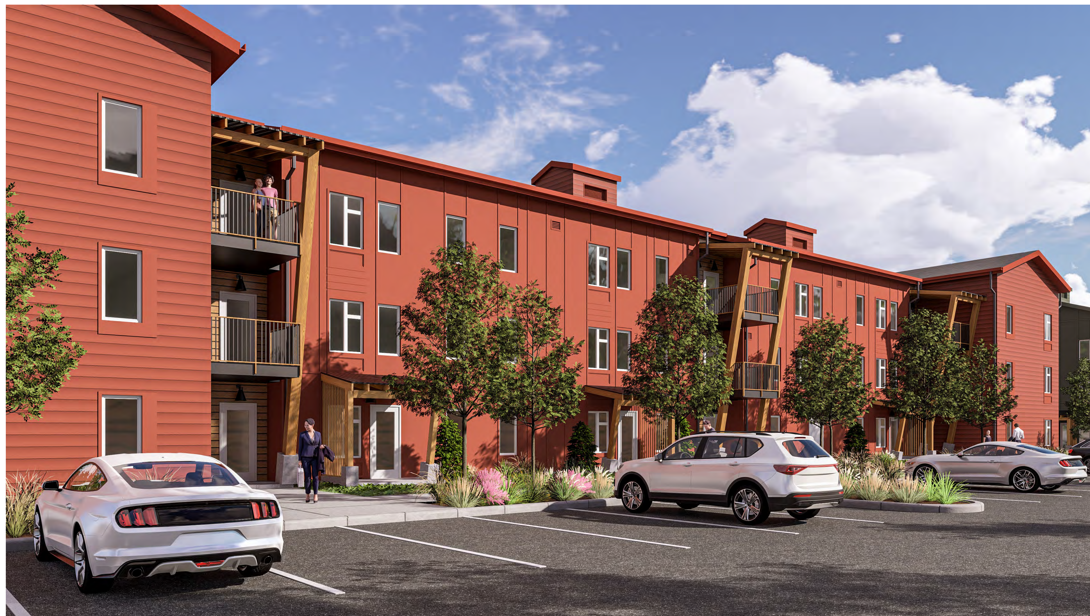
BUILDING 1 - LOOKING SOUTH
