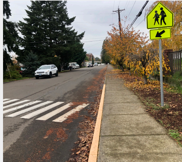
There are two high-visibility crossings on 7th St. However, curb ramps are needed to facilitate access at these crossings.
