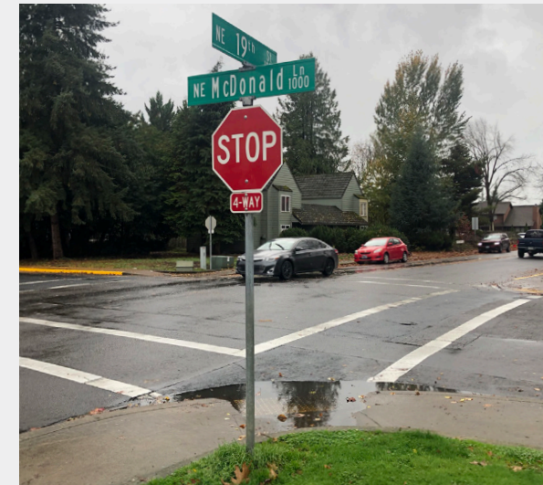
19th St and McDonald Ln is a heavily-utilized four-way stop at the southwest corner of the campus. This crossing does not have adequate lighting during the winter months, and it lacks high-visibility crosswalk markings, which could help with visibility.
