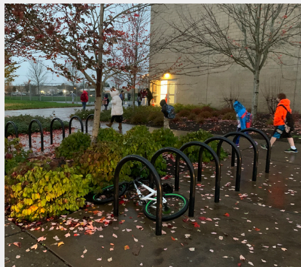
Bike parking is provided, but is not covered. During rainy or windy weather, bicycles are not protected.
