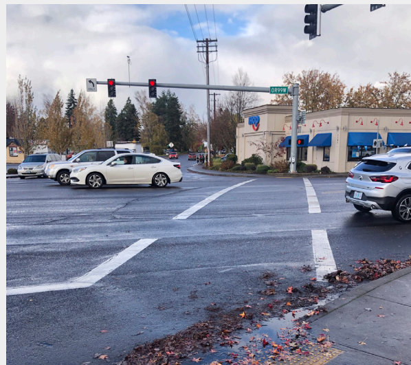
The crossing of Hwy 99 at McDonald Ln is one of the more hazardous crossings for students. Some reported feeling uncomfortable when traveling through this intersection.
