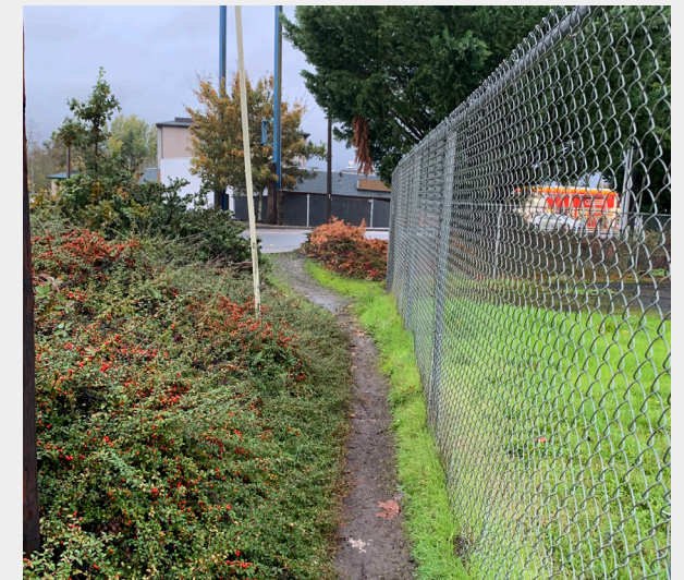
The approach to the NE corner of Booth Bend Rd and Hwy 99 lacks an accessible sidewalk and is overgrown with vegetation.
