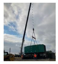
To provide actual redundant power, two generators were installed. One at the Water Reclamation Facility, and the other at the Raw Sewage Pump Station (RSPS).
