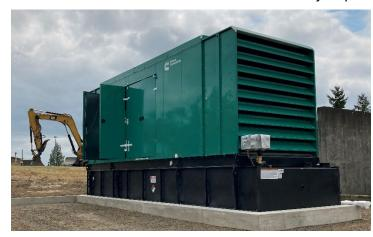
The City continued to invest in upgrades to the public sanitary sewer system in 2021. Work included installation of 1000 KW generators at the Water Reclamation Facility and the Raw Sewage Pump Station.
