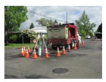
7,355 feet of mainline pipe was rehabilitated using Cured In Place Pipe (CIPP) lining.
