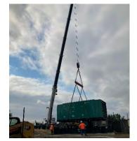
The final generator needed to complete our redundant power requirements at our pump stations will be installed this year at our Cozine Pump Station.
