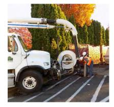
*Conveyance Systems crew cleans a sanitary storm line using one of the City's vacuum trucks.*
