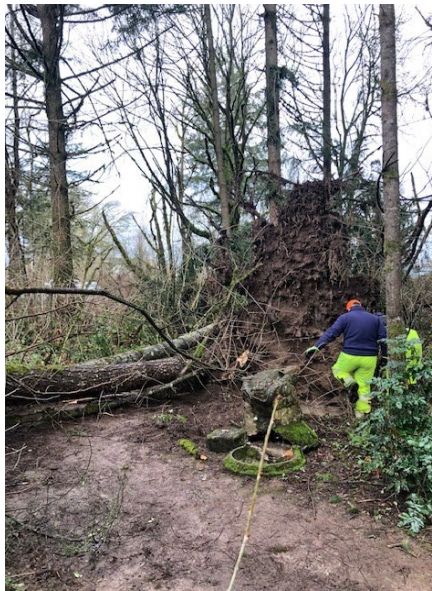
Parks Maintenance crew surveys damage at Airport Park after a day of high winds.
