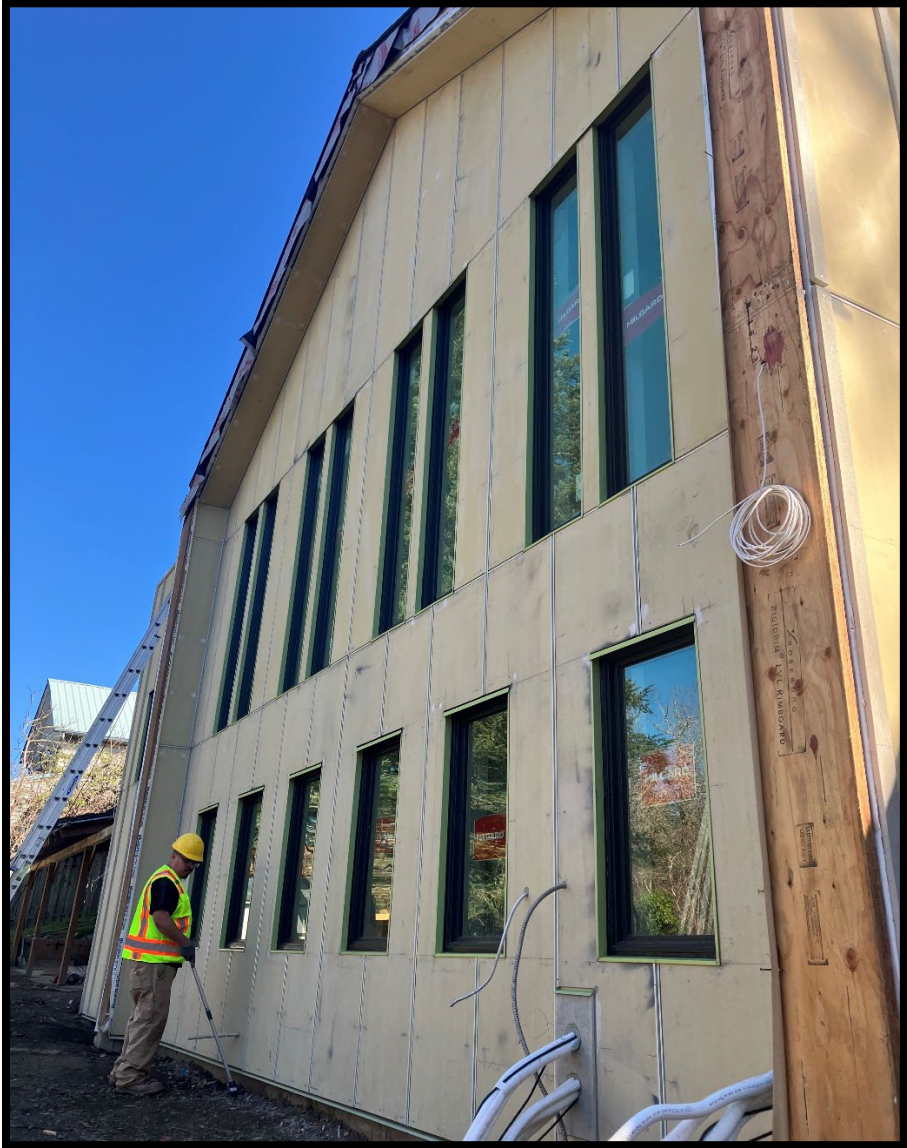
Construction of the new Navigation Center (Low Barrier Emergency Shelter)
