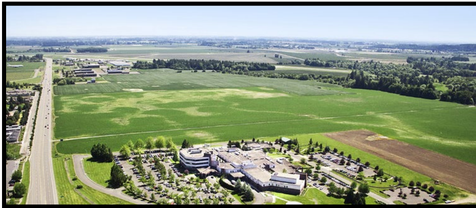
Innovation Campus Site
