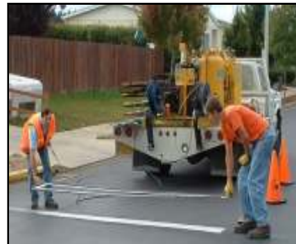
Thermoplastic traffic markings are replaced as necessary, and each stop sign in the system includes a stop bar. Staff replaces approximately 1,000 lineal feet of markings and applies yellow paint to approximately 5.5 miles of curb each year.
